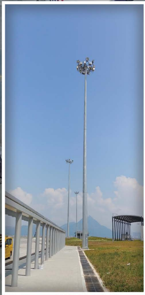
HM Hong Kong Zhuhai Macao Bridge Vehicle Clearance Plaza - Abacus High Mast
