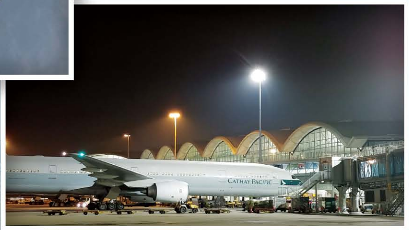
HM Hong Kong International Airport - Schreder Omnistar LED Floodlight
