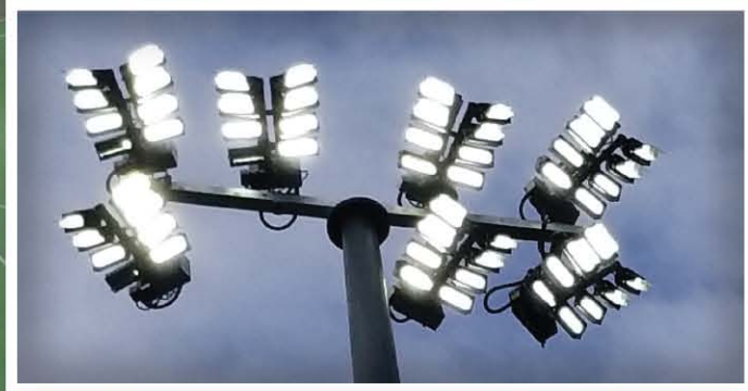
SL Jockey Club HKFA Football Training Center – Abacus High Mast & LED Floodlight
