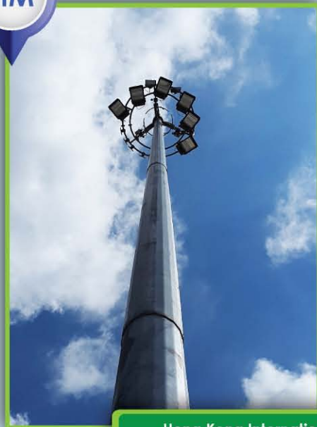
Hong Kong International Airport
