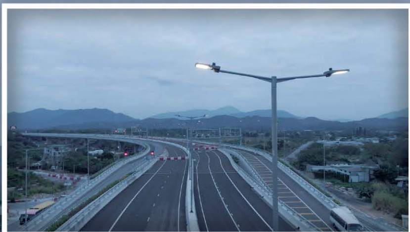
RL Heung Yuen Wai Highway – Schreder Avento LED Road Light
